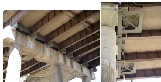
US40/I64 in St. Louis, MO retrofit with restrainers and seat extenders
