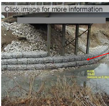
Gabions for scour protection
