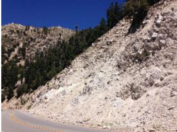
A highway slope exposed to rockfalls
