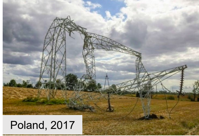
Tower rupture-windstorm
