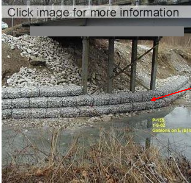
Gabions for scour protection
