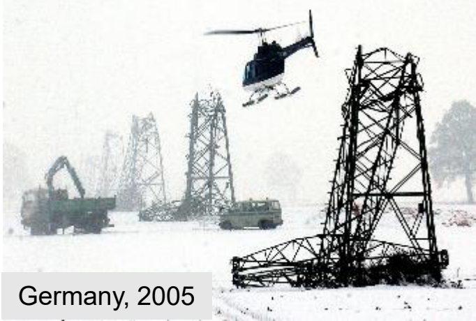
Tower rupture-snowstorm
