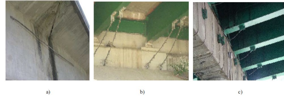
Fig. 9. Restrainer cables (a) in Kentucky connecting two adjacent girders; (b) in Tennessee (SR59 over I-40) connecting girders to the abutment; and (c) in Illinois attached to girders and wrapped around bent beam
