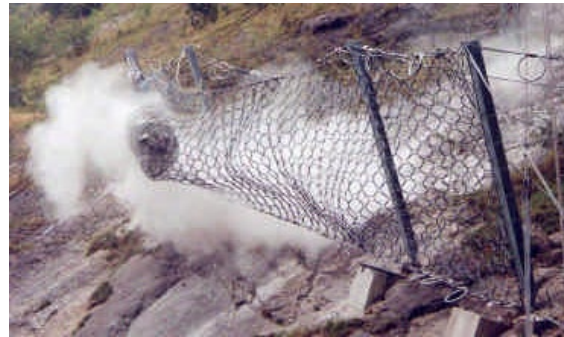
Protection barriers during rockfall event
