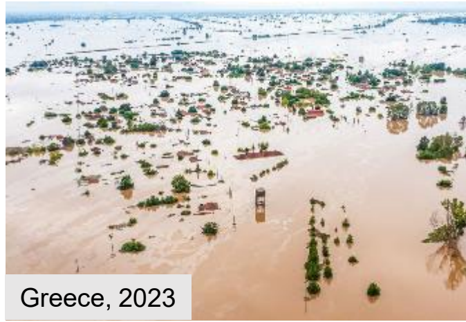
Substations and towers-flood
