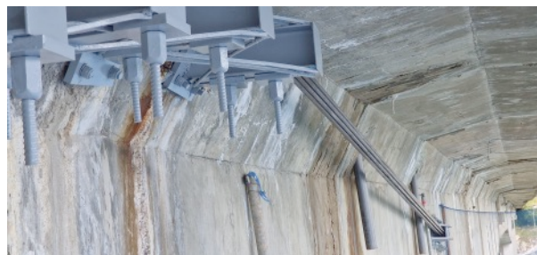
Intervention on the most critical half joint
