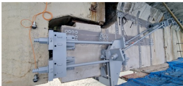
Intervention on the most critical half joint
