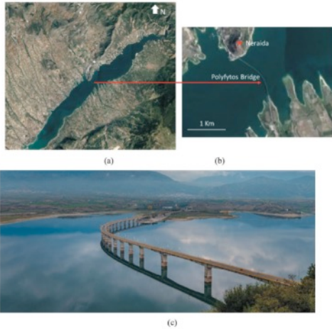
Figure 1. The landmark Polyfytos Bridge: (a) Polyfytos bridge wider area (b) focus area (as obtained by Google Maps 2020), and (c) panoramic view of the asset with the precast spans (direction Kozani-North to Servia-South) and the long spans with the cantilevers in question at the bottom right side of the photograph.
