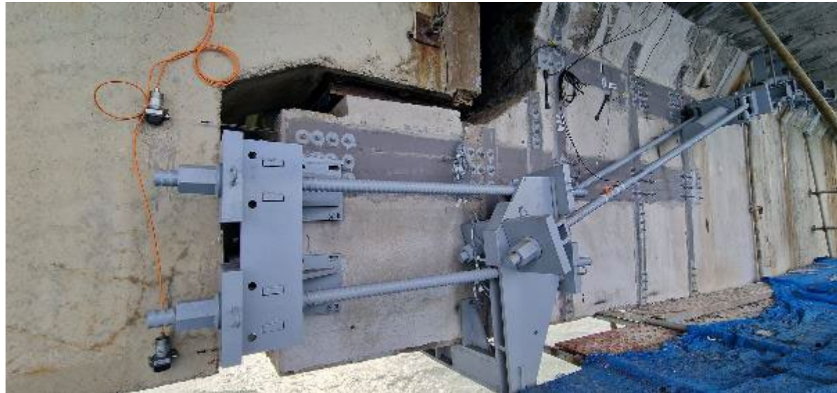
Intervention on the most critical half joint
