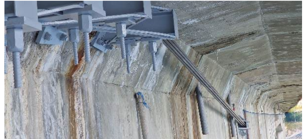
Intervention on the most critical half joint
